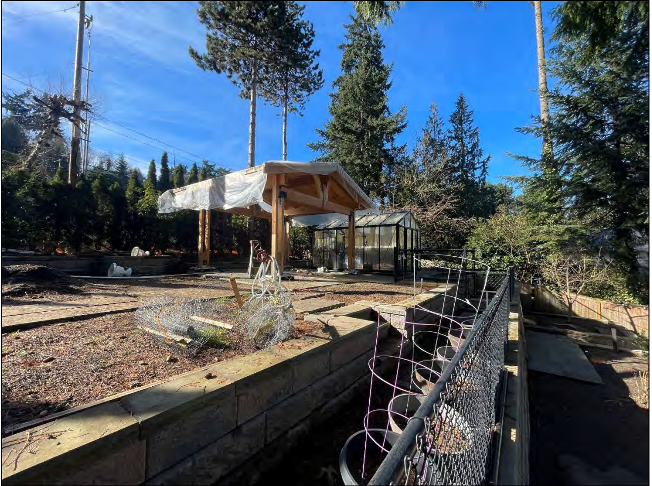
Photo 3. Looking southwest toward recent site work.
